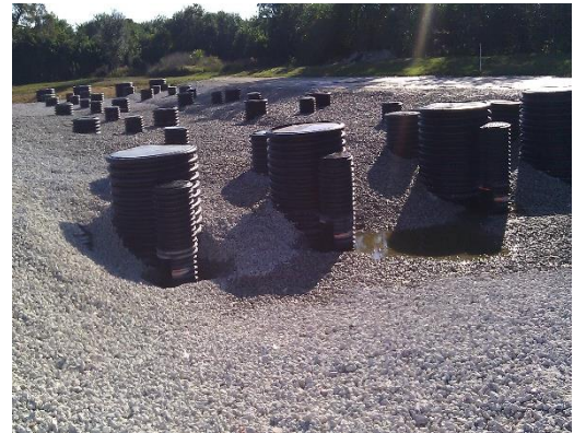
Fig. 1.10 Anaerobic Zone (Rock) and Upflow Filter (Pipe)
