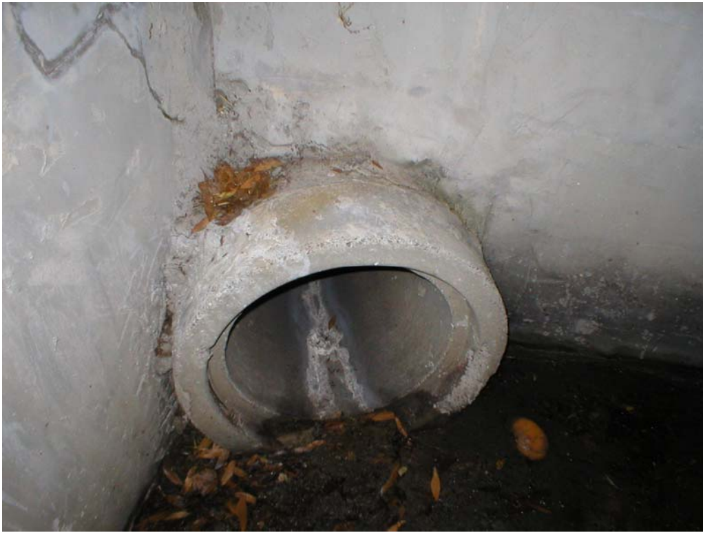
Figure 7. Inside AD2 - inlet in Basin 2. Note leaf and grass loads.
