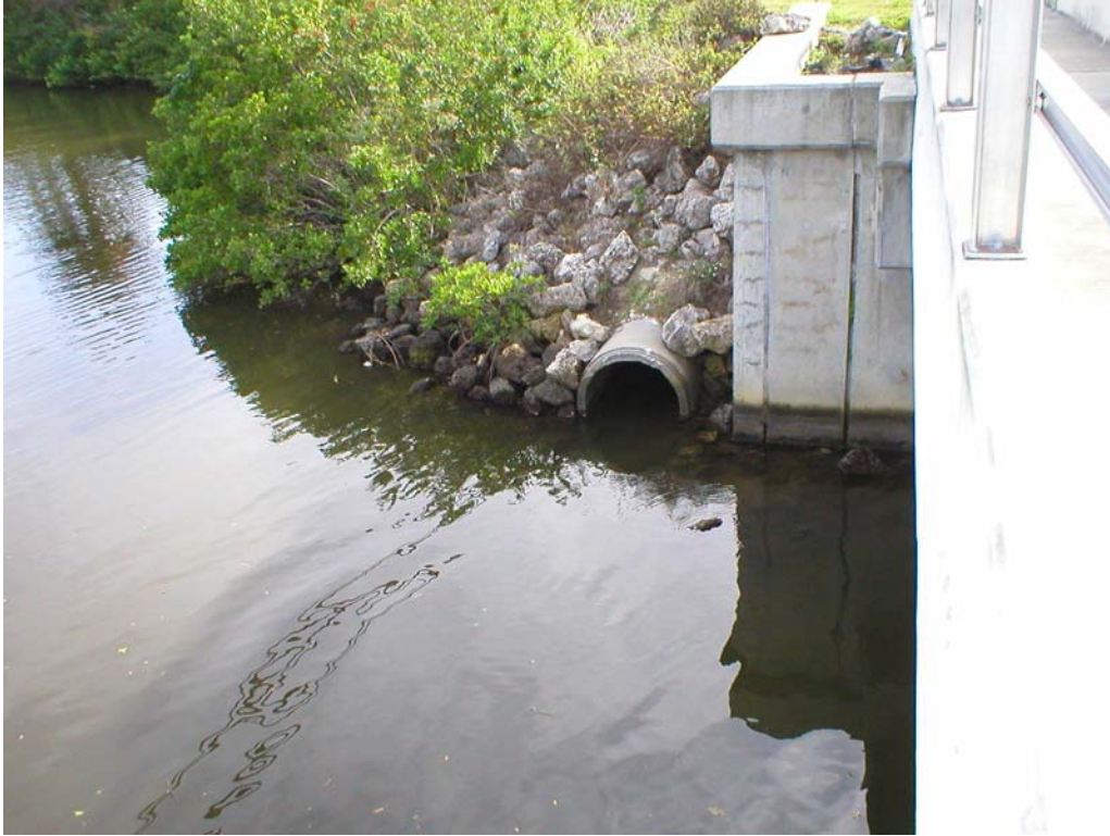
Figure 16. Outfall AD8 at base of US 41 bridge.
