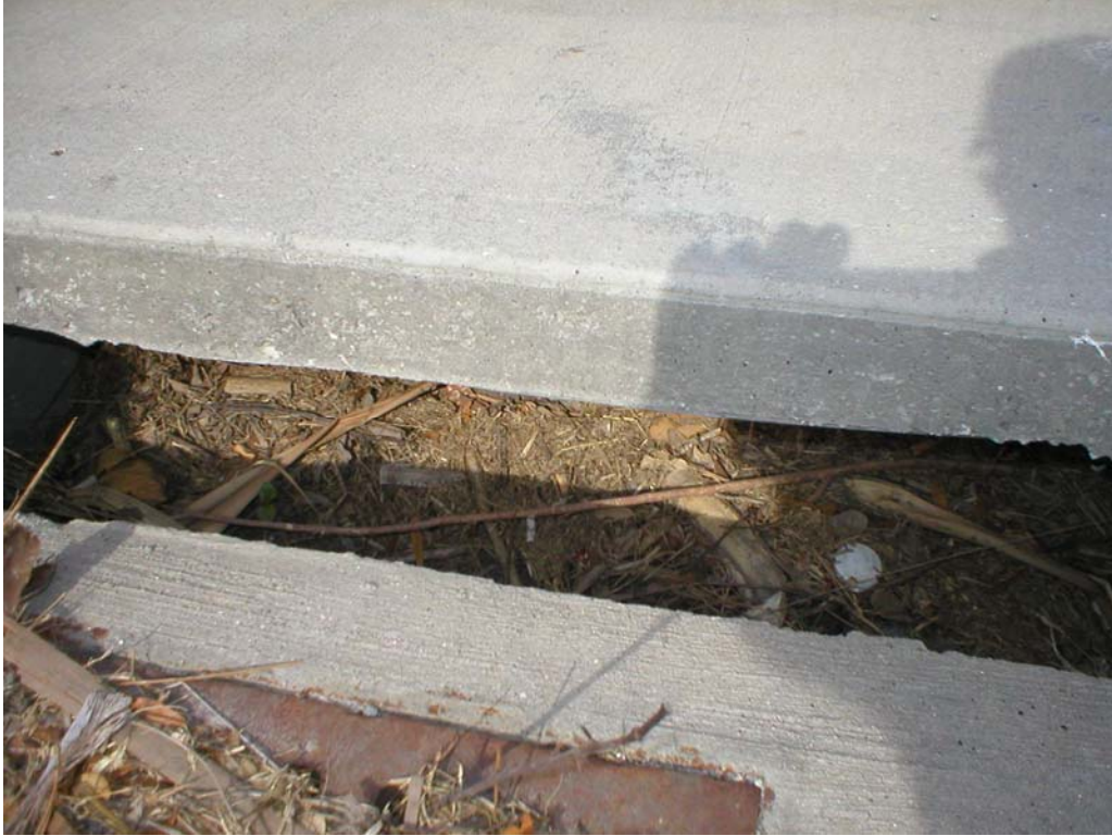
Figure 11. AD5 - Inlet clogged with leaves and debris in Basin 5.
