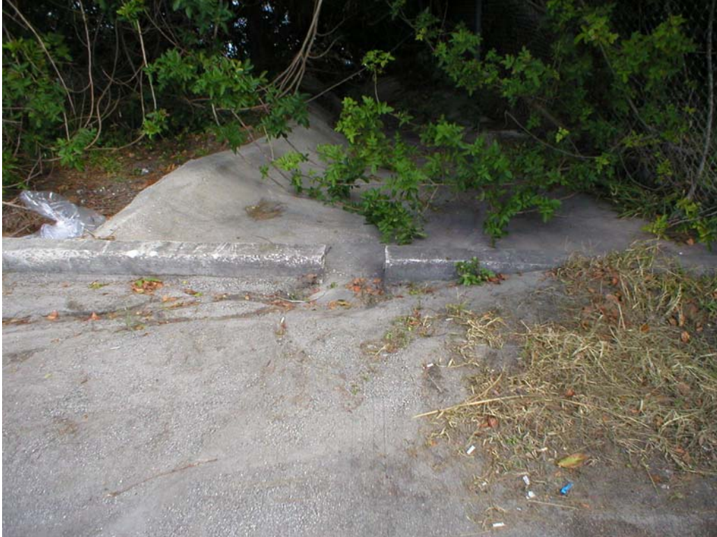
Figure 13. AD7 – Curb cut in Basin 7. Note sediment build up next to curb.
