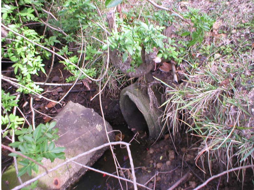
Figure 5. Outlet AD1 in Basin B1. Note culvert lying in canal and steep bank erosion.
