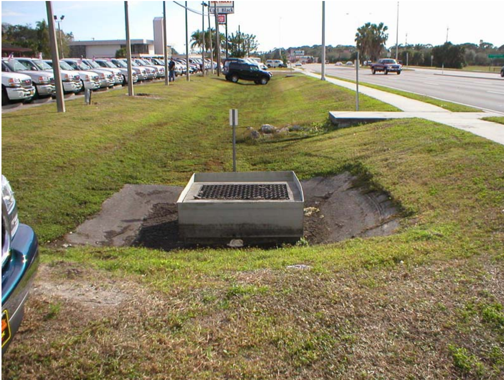
Figure 15. AD8 - Roadway swales and raised inlet along US 41.
