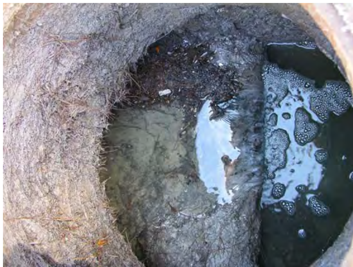
Figure 10. Sediment and organic debris within the Beach Road stormwater pipe system.
