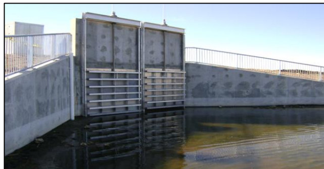
Flood Gate between South Cell and Walker Tract
