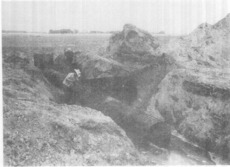
Figure 3. Installation of this gravity drain took place May 16, 1967.
