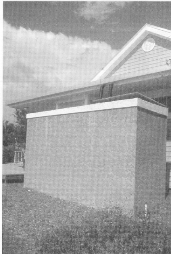
◀ Rain gutters connected to large concrete cisterns can collect and hold thousands of gallons of rainwater that can be used for irrigation or flushing toilets.
