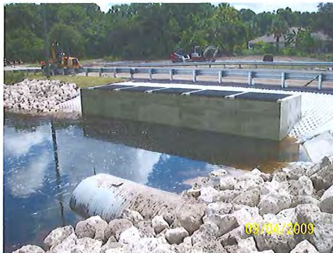
Newly constructed Water Control Structure #503 on Apollo Waterway with fiberglass skimmer to prevent clogging and triple 72" concrete culvert pipes under Chancellor Blvd through a cooperative joint project with Charlotte County Public Works
