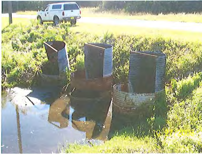
Old Water Control Structure #503 on Apollo Waterway - Note corroded metal drop pipe design which is subject to clogging
