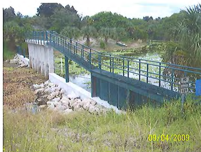
Newly retrofitted Water Control Structure #109 on Cocoplum Waterway with concrete weir and 6 new stainless steel gates
