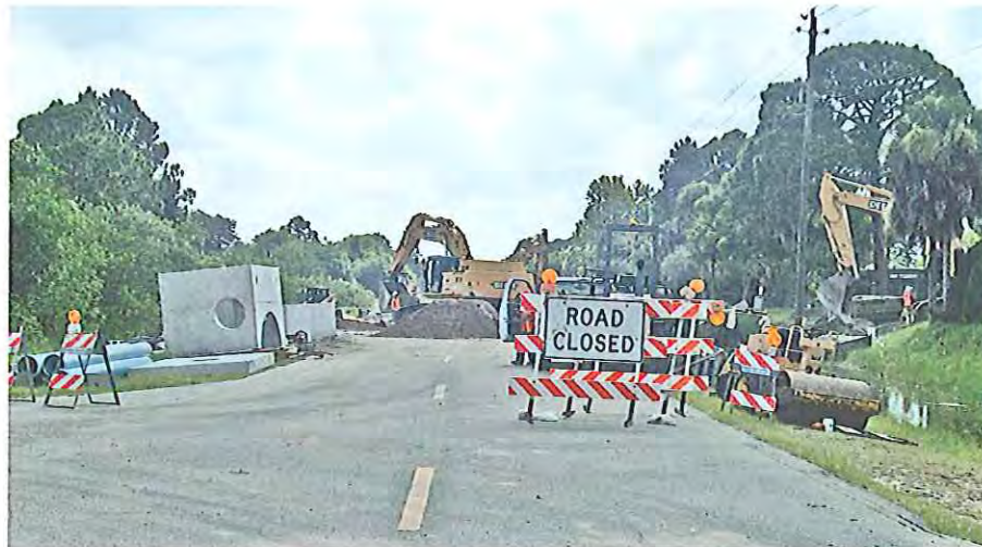
Water Control Structure #501 on Cheshire Waterway – Replacing concrete structure and 60" diameter corroded metal pipe with concrete pipe
