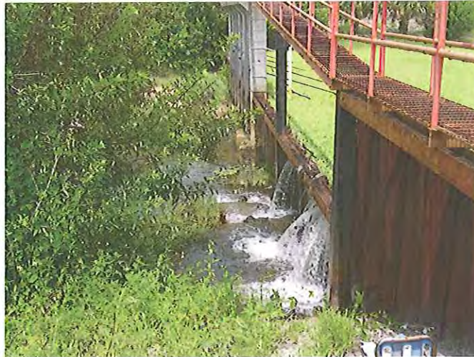
Old Water Control Structure #109 on Cocoplum Waterway with corroded metal weirs and 6 corroded gates. Note water pouring through large holes in the corroded metal weirs.
