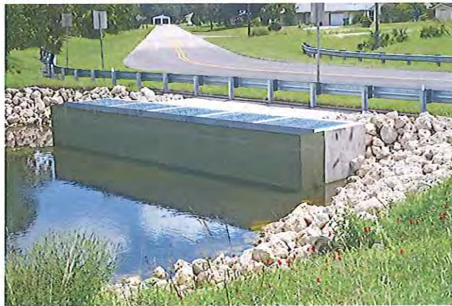
Newly constructed Water Control Structure #504 on Jupiter Waterway with fiberglass skimmer to prevent clogging and triple 72" concrete culvert pipes under Chancellor Blvd through a cooperative joint project with Charlotte County Public Works
