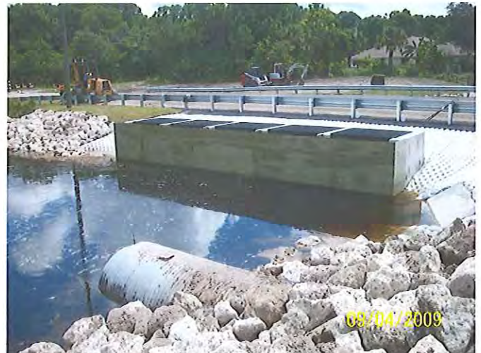
New Water Control Structure #503 on Apollo Waterway
