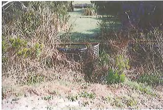
Old Water Control Structure #504 on Jupiter Waterway - Note corroded metal drop pipe design which is subject to clogging
