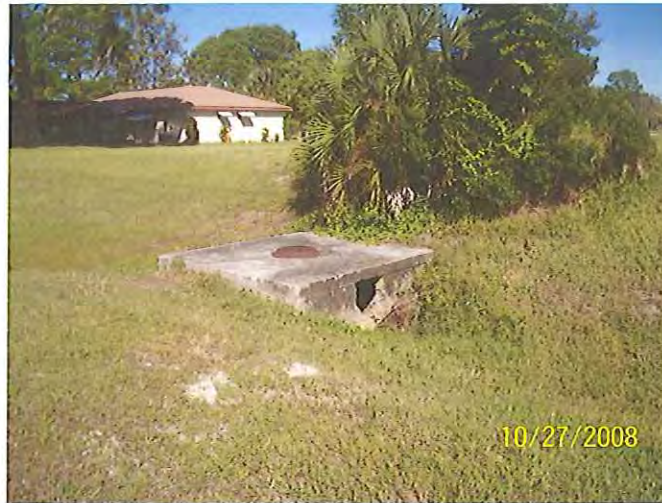
Old Water Control Structure #501 Discharging into Cheshire Waterway – 60" metal pipe connect to this concrete structure is corroded under Chancellor Blvd
