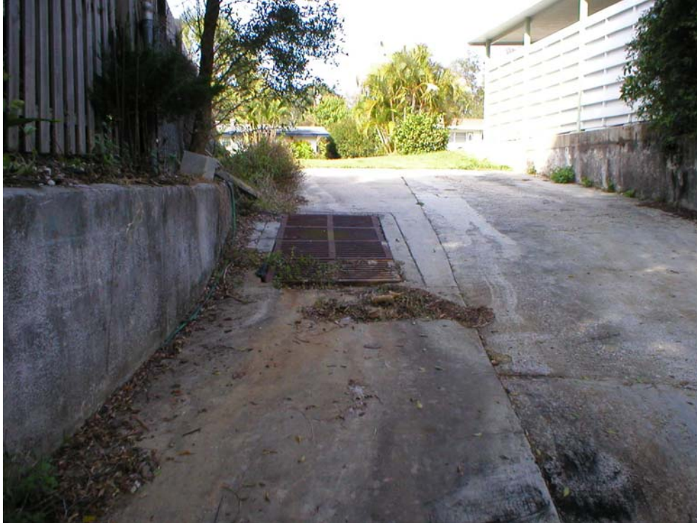
Figure 13. PC3 outlet discharges through a grate on the boat ramp.
