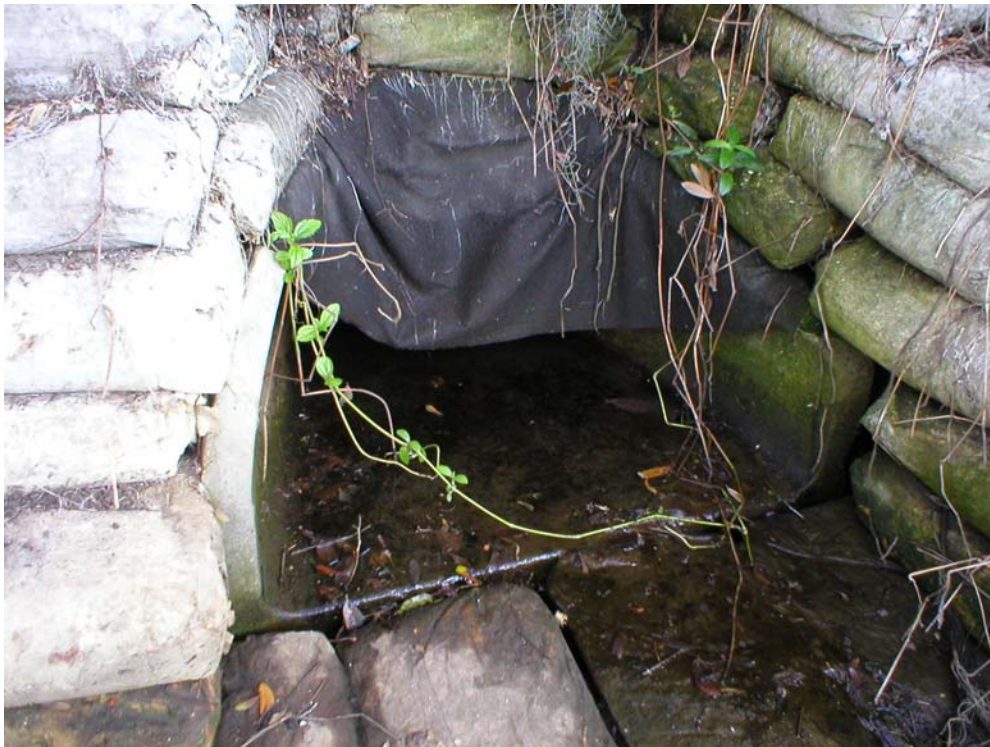
Figure 11. PC2 outlet mitered end. Note thin layer of muck.
