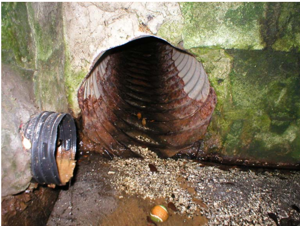
Figure 5. Inside inlet PC1. Note sediment loads.
