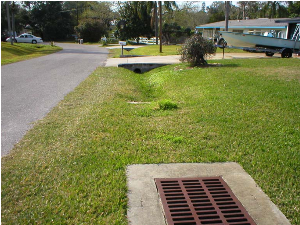
Figure 12. PC3 inlet with diversion structure in Basin B3.
