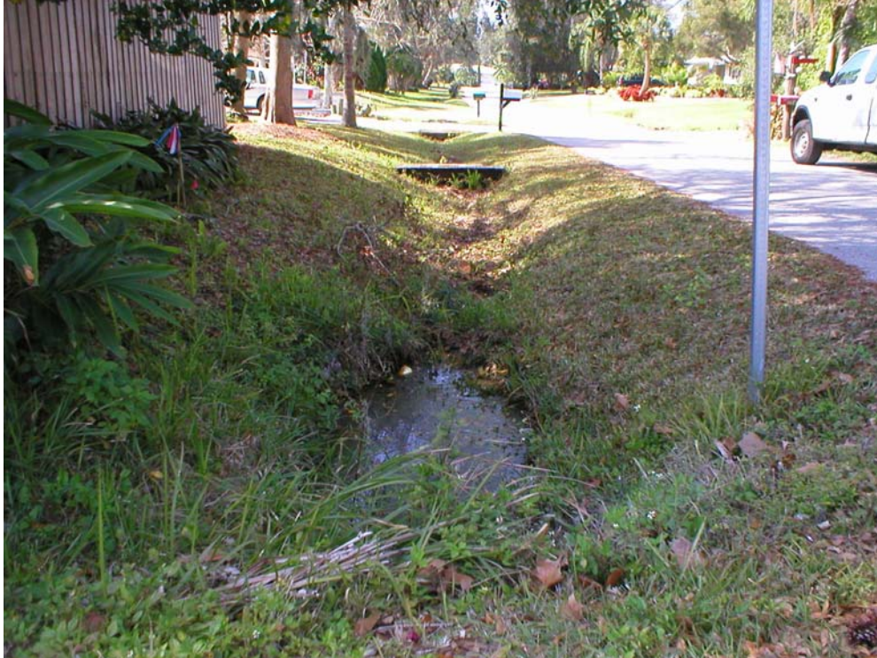
Figure 10. Swales along Trinidad St. upstream of PC2.
