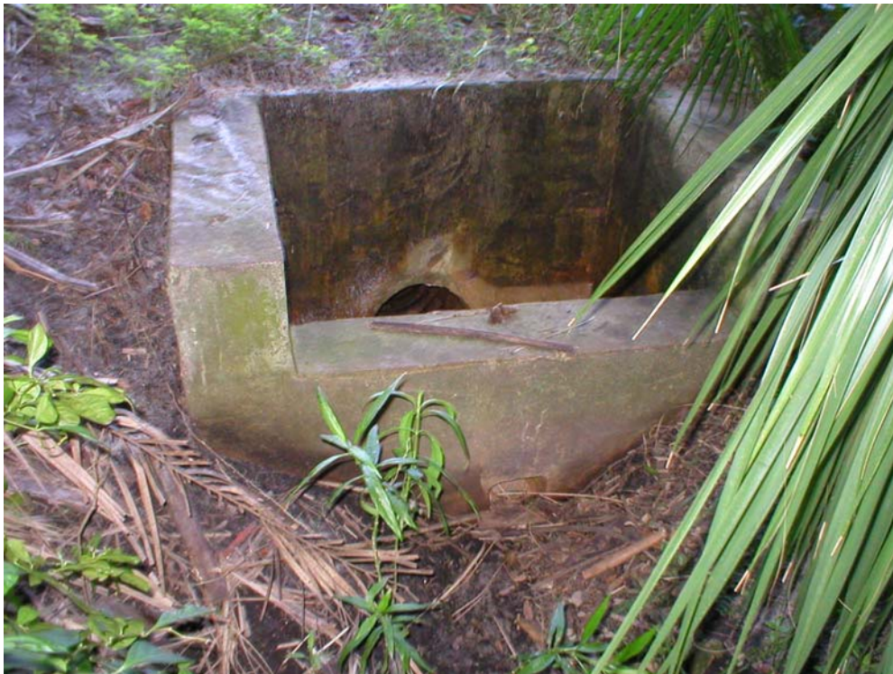
Figure 7. Outlet structure at the end of the swale on PC1.
