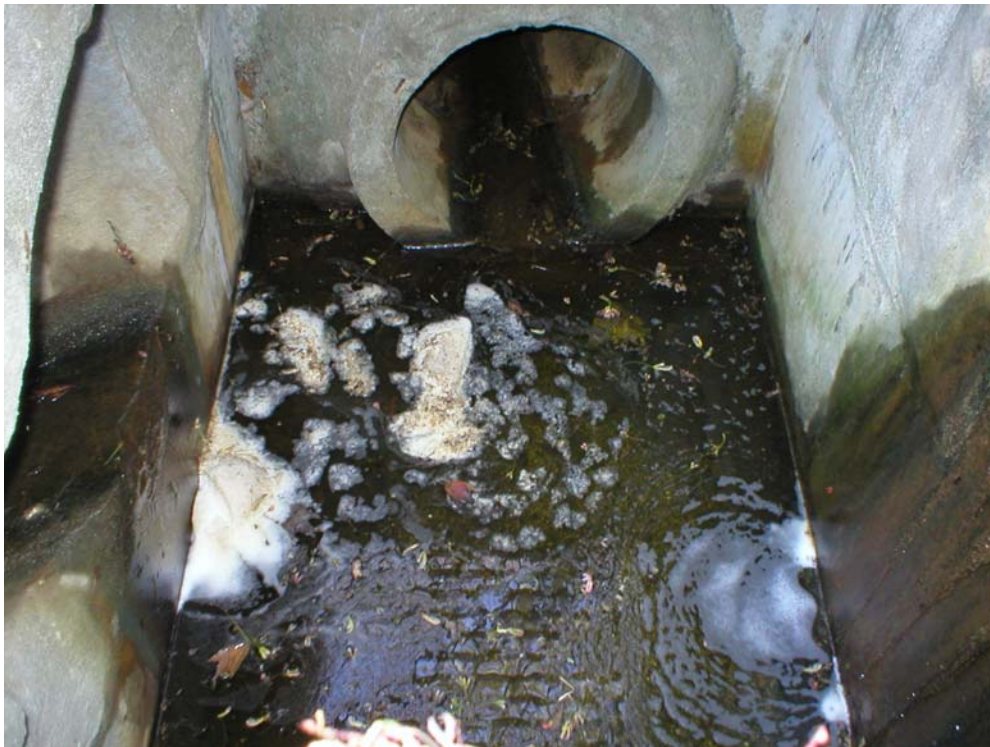
Figure 9. Inside inlet PC2. Note foam floating at the bottom of the inlet.
