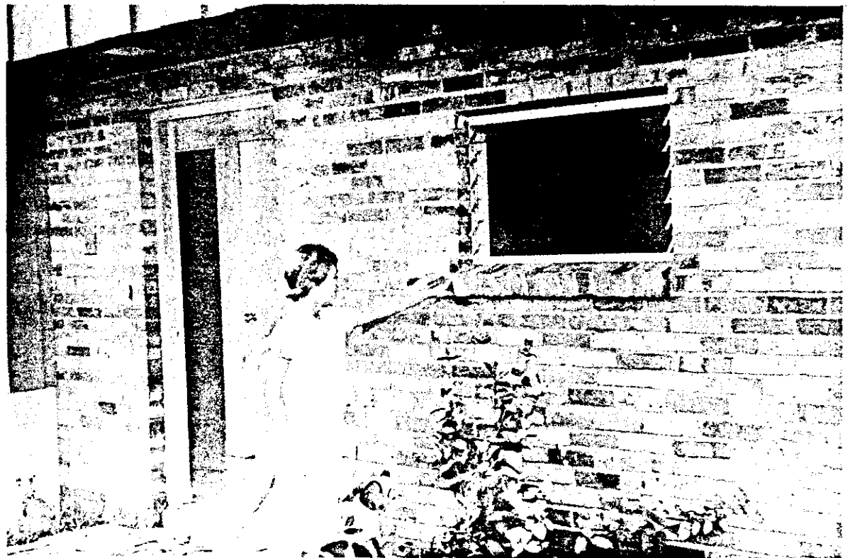
PHOTO 16. HIGH-WATER MARK, ABOUT 5 FEET ABOVE GROUND, ON SARASOTA HOME IN BELLEVUE TERRACE. (SEPT. 1962)
