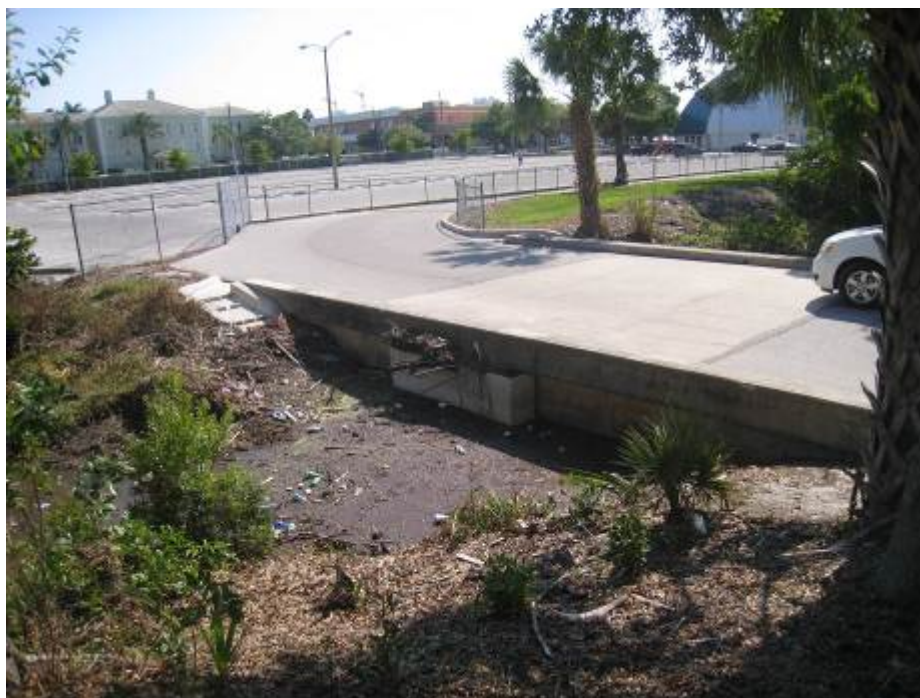
Figure 8-39 Skimmer and Culvert to East Branch of Hudson Bayou, Facing Southwest
