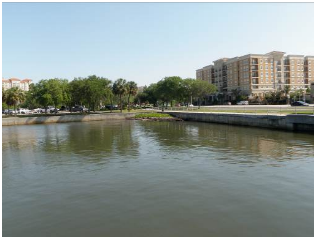
Figure 8-33 10 th Street Boat Basin, Northeast Corner
