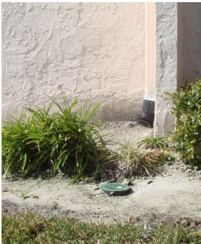
Figure 8-43 Rain Gutter Bubbler System
