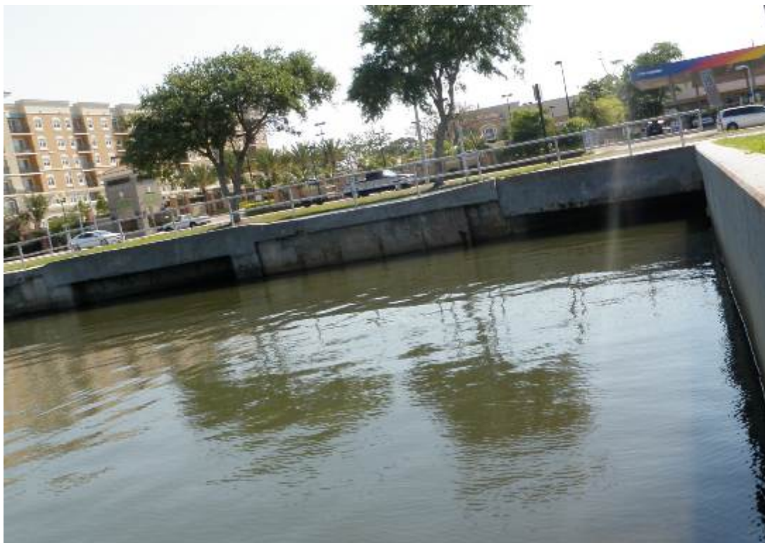
Figure 8-32 10 th Street Outfall
