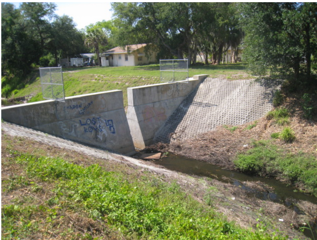
Figure 3-18 Weir in Hatton Street Ditch, Facing Northwest
