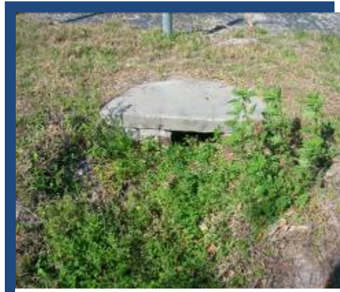
Photograph 38 Drop Inlet Structure at West End of Ditch
