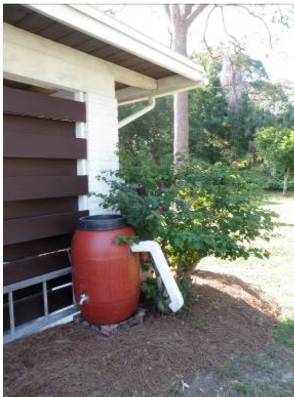
Figure 8-42 Rain Barrel System
