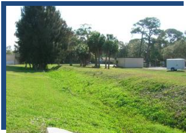
Photograph 36 Facing East of Ditch at South End of Park
