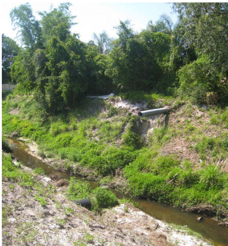
Figure 3-17 Outfalls to Hatton Street Ditch
