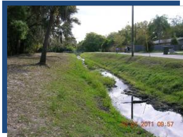
Photograph 24 Facing East of Ditch at South End of Park Flowing East
