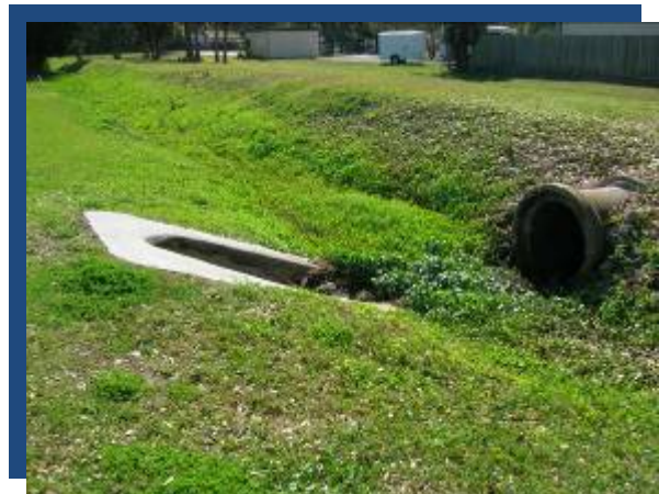
Photograph 37 Inlet Pipes from East Pond (Left) and Apartment Complex (Right)
