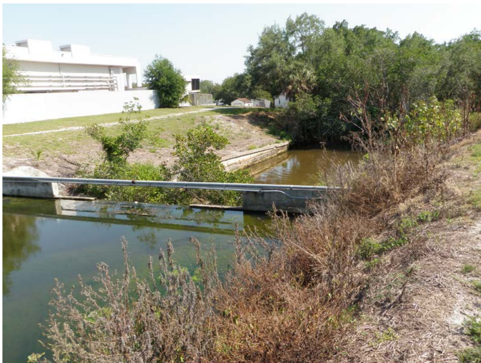
Figure 3-21 Site 7, Facing South
