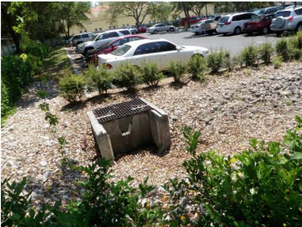
Figure 8-25 Site 5 Outfall at North Side of South Lot
