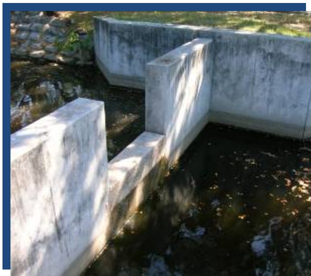
Photograph 4 Weir at South End of Pond
