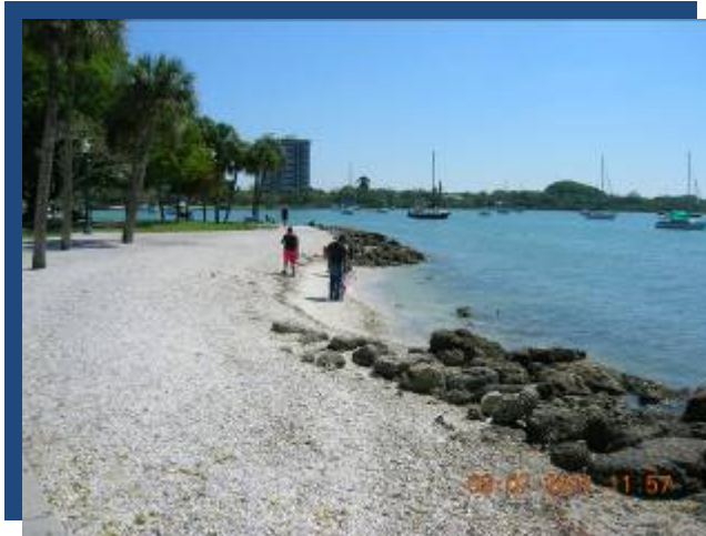
Photograph 11 Shoreline Rock Armor along West Tip of Park
