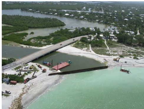
View after dredging and just prior to removal of the retaining wall
