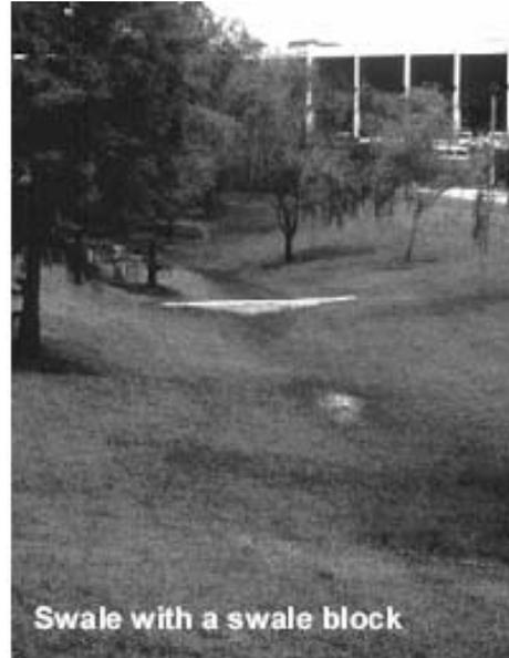
Ponding of runoff in the swale allows the water to soak into the soil, helping to reduce the volume and amount of pollutants.
