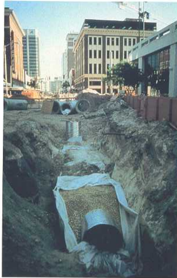
Orlando Streetscape Project Exfiltration Trench
