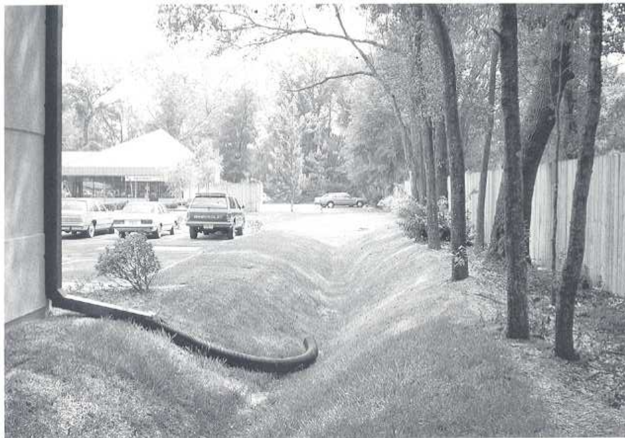
Infiltration Practice: Directing roof runoff to grassed areas.
