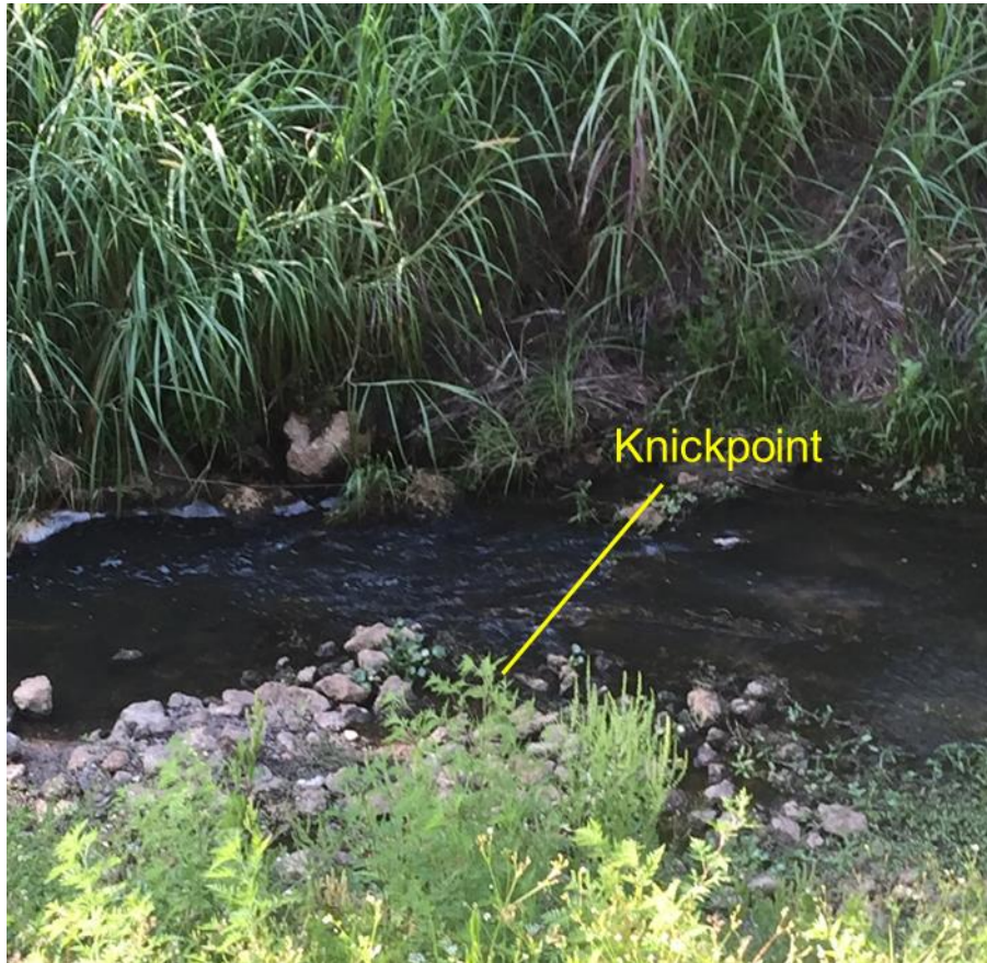
Figure 5. Degradation with Migrating Knickpoint (Canal 15).
