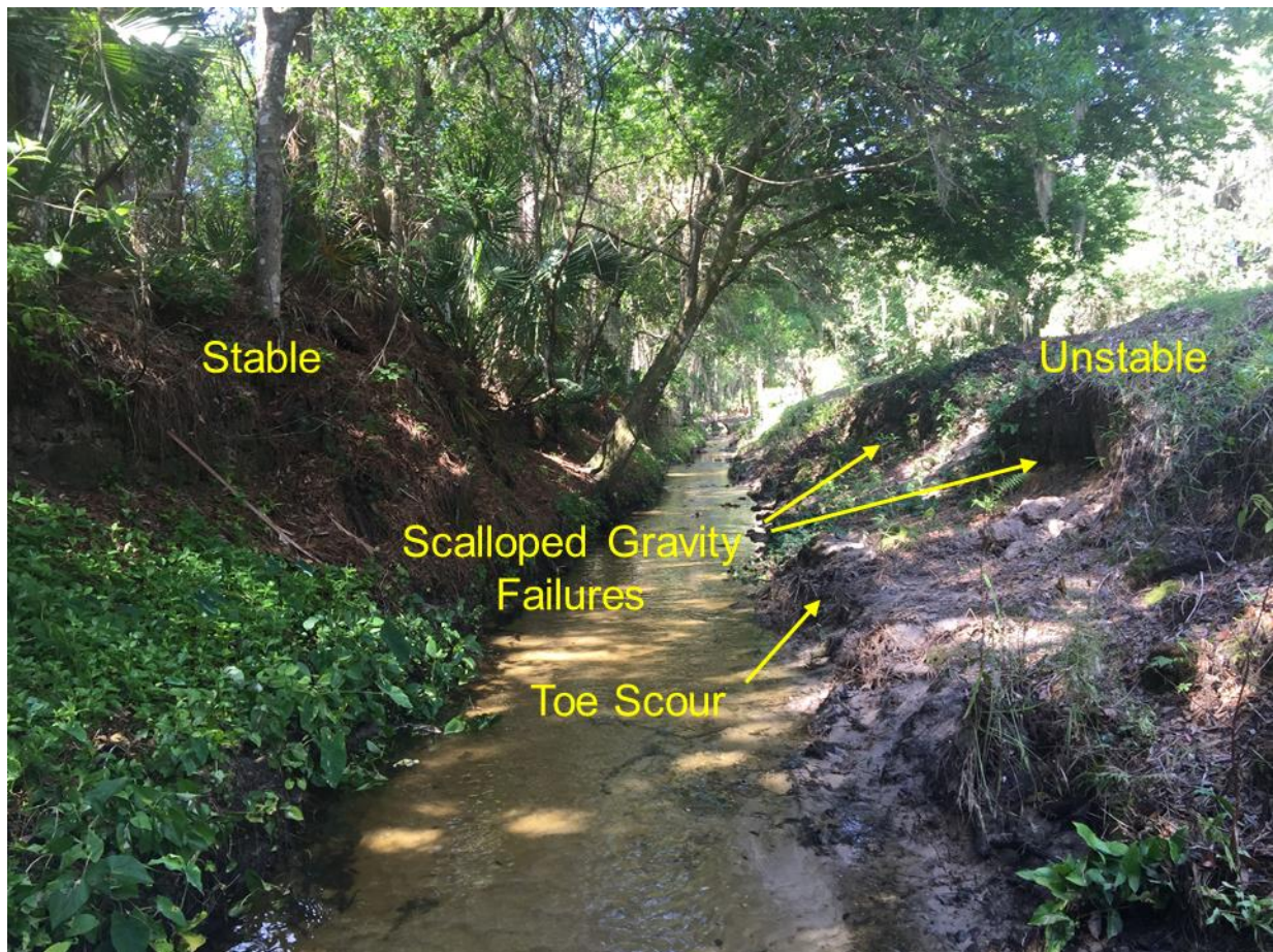
Figure 2. Stable Woody versus Unstable Non-Woody Banks (Canal 302).
